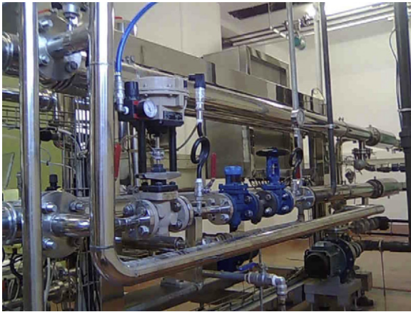
Fig. 2. Electropneumatic globe valve.
